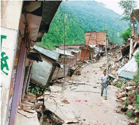
Photograph-3 ; Slumping Of Shops In Bhatwari (2013)
