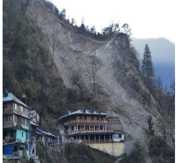
Photograph-6 ; Gangnani Landslide(2016)
