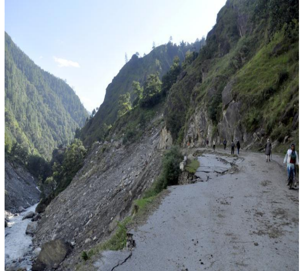
Photograph-5; Landslide Near Sunagarh(2016)
